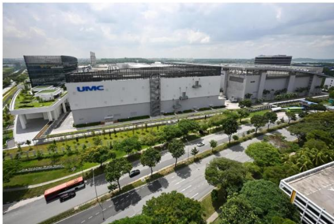
UMC's new plant (left), which is next to its existing fab facility, will take its annual production of integrated circuit wafers to 1.3 million in the next few years. ST PHOTO: LIM YAOHUI
